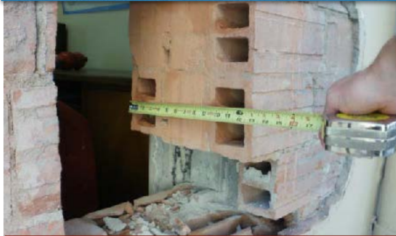
Cut into walls to measure thickness
